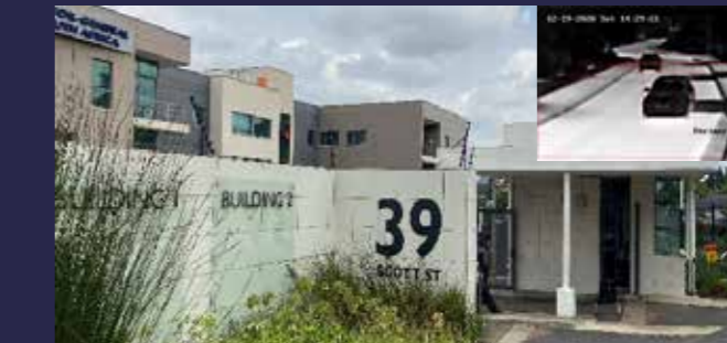
Office Building Entrance
